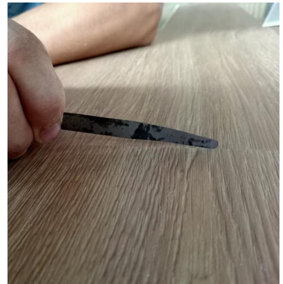
Joint Seam check
